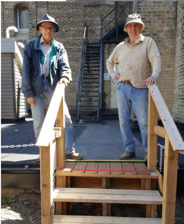
Don and Chuck with upgraded access steps for boiler roof walkway.
