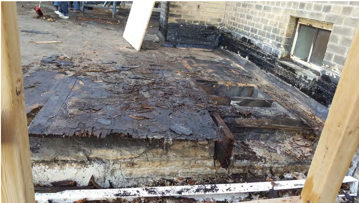
Removing old boiler roof, repairing rotted wood. 7 May
