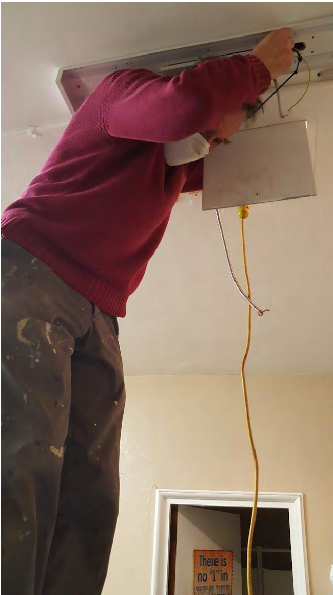
David Wilcox replacing a fluorescent ceiling fixture with LED.
