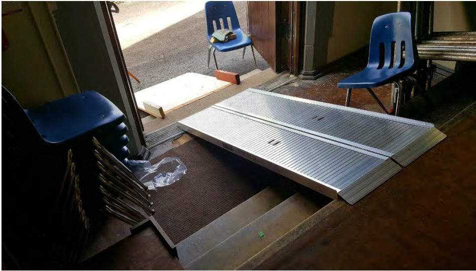
Accessible exit ramps from Sanctuary at NW exit to driveway.
