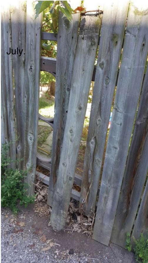
Left: boards falling off the fence alongside the driveway in
