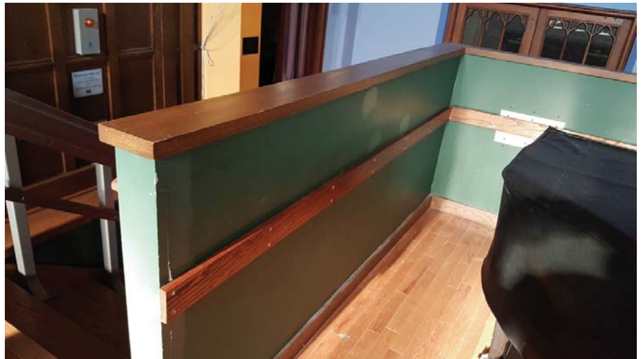
Below: the new 'rub rail' to protect the drywall from the careening grand piano.
